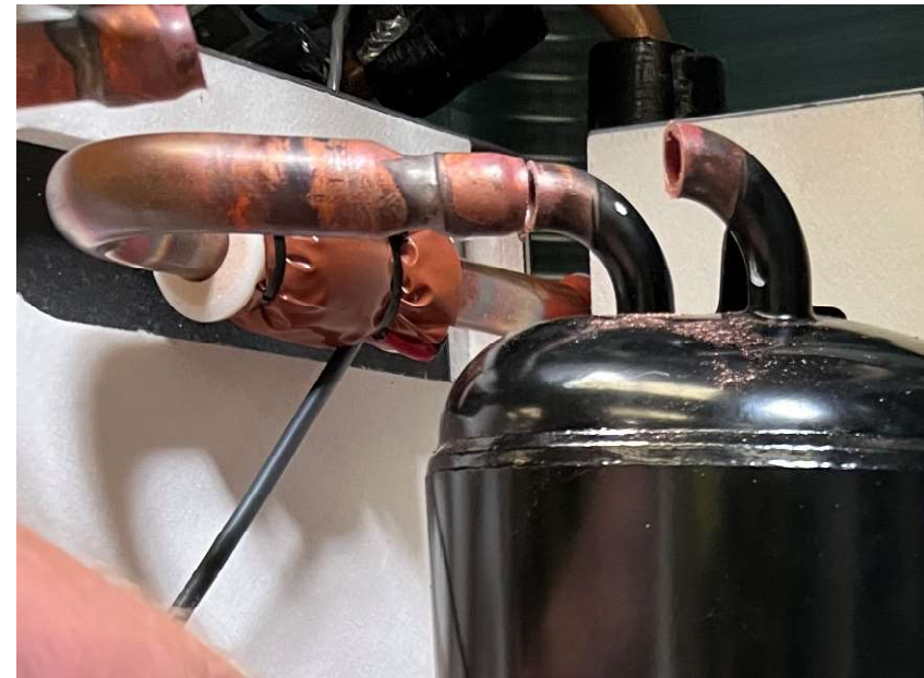
Cutting process of the compressor without flame
